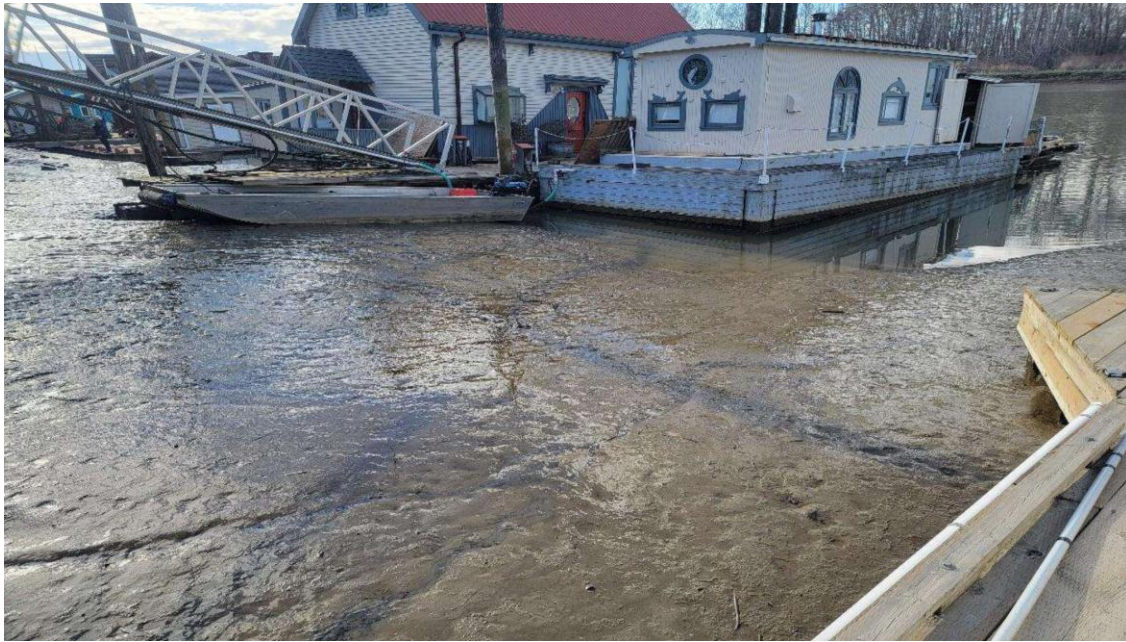
Silt Accumulation within Ladner Harbour
